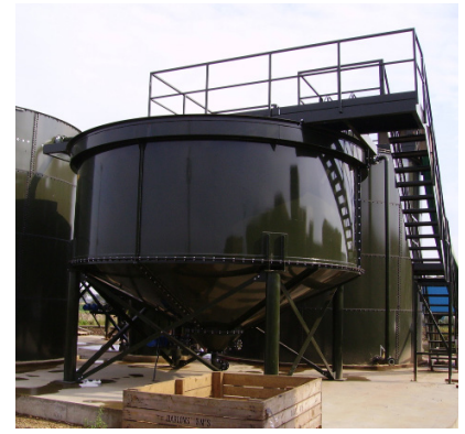
Liquid Tank Level Monitoring
