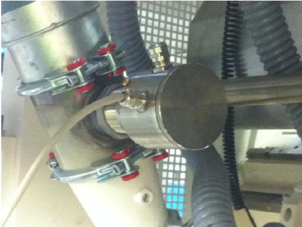
Flow monitoring system FS 510 mounted on the edge trim extraction
